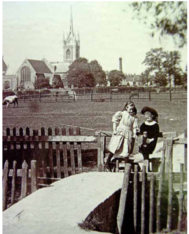
The Cooksditch bridge over Faversham Creek (1895) © The Faversham Society
