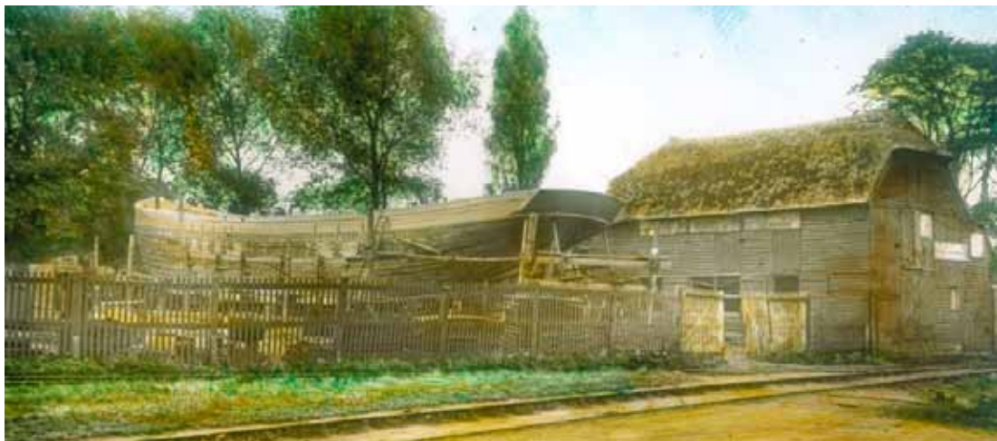
The launch of the concrete ship Molliette, 1918 / A sailing barge being built by the creek © The Faversham Society
